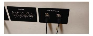
The leads that plug into the wall sockets plug in to the mixing deck using the Main Out ¼ inch sockets in the top-right corner of the
