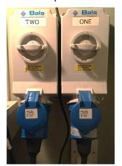
floor on the right-hand side of the lighting cupboard. The two packs give a total of 12 channels for halogen lights so each 15amp plug can occupy a numbered bank (each bank actually has two sockets but we only use one plug per bank to give more control). Each dimmer pack has a 32amp mains plug which needs to be plugged into
