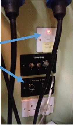
Sound can be input to the deck from an external source such as a computer or headphone socket of a tape player. In the picture below this has been done this using channels 11/12 with a converter lead from 3.5mm stereo jack to ¼" Mono Jacks. (you must supply these external leads/connectors for your equipment).
