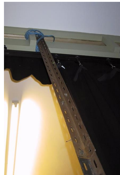
Figure 2 - Side flat Dexion attached to village hall curtain rail
